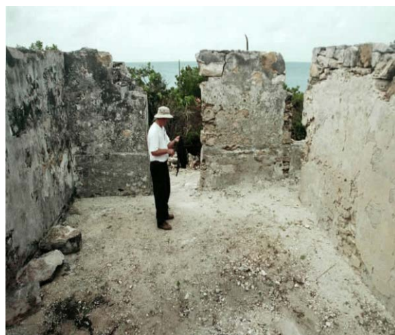
Figure 6. The central room looking to the West through the middle door. Full height of the wall remains. Interior has been shoveled out.
